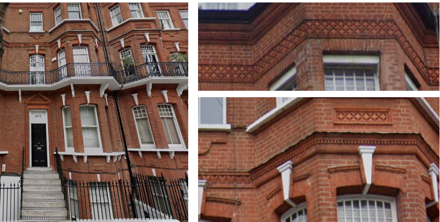
Photography of architectural details of 7-27 Tite Street
