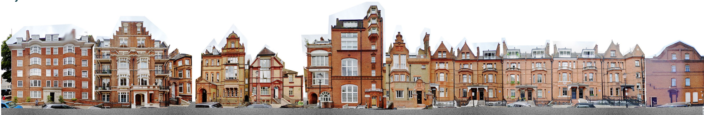
Photo montage of 26-58 Tite Street.
